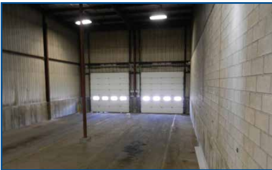
Overhead Doors to Warehouse Building #5
